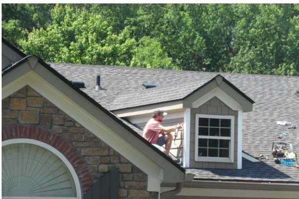
Rotten dormer boards were replaced and repainted after new roofs were installed on the units.
